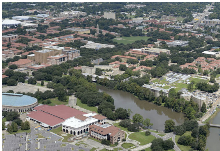
CAMPUS FLOODING AUGUST 2016
