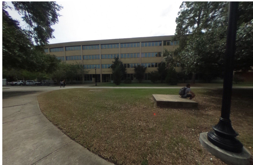
EXISTING HISTORIC QUAD
