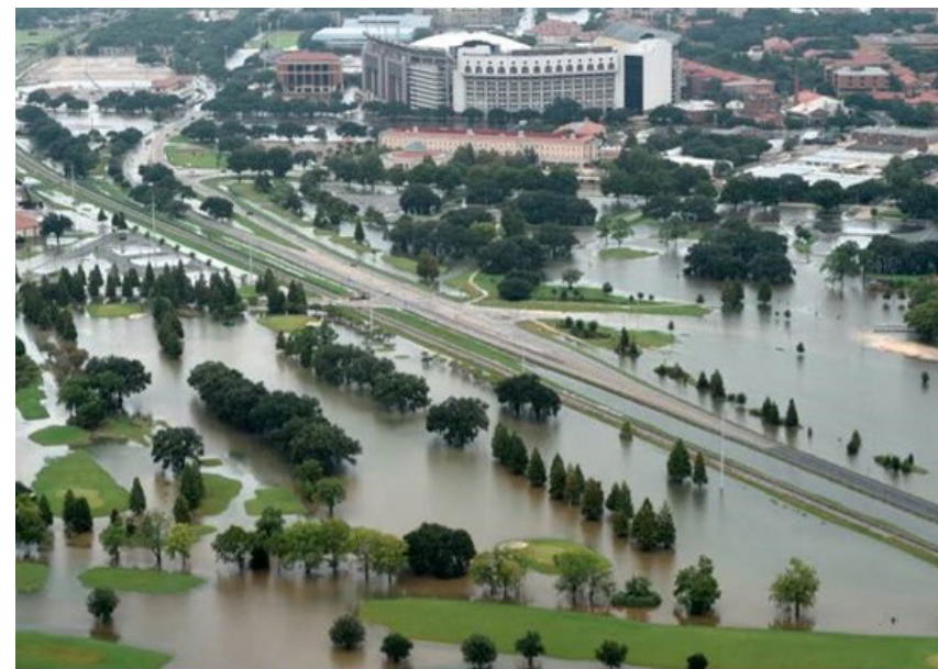
CAMPUS FLOODING AUGUST 2016
