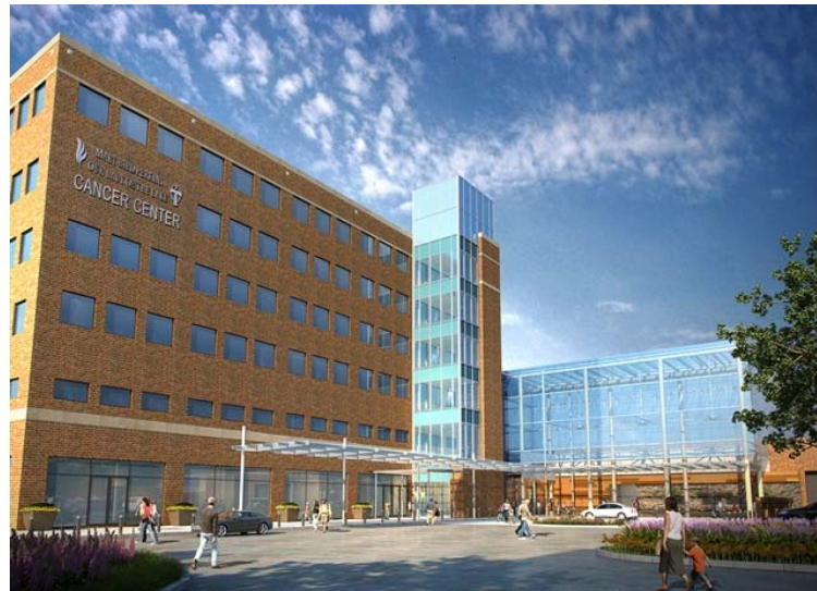
Front view of MBPCC when renovations are complete
